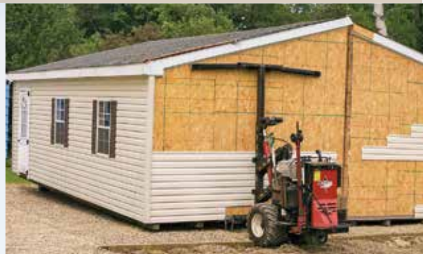
Moving a modular garage into position
