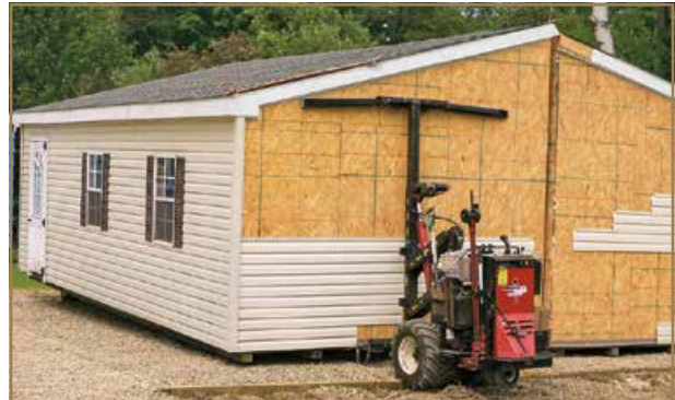
Moving a modular garage into position
