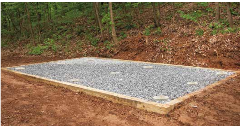
10x12 shed pad with concrete pillars
