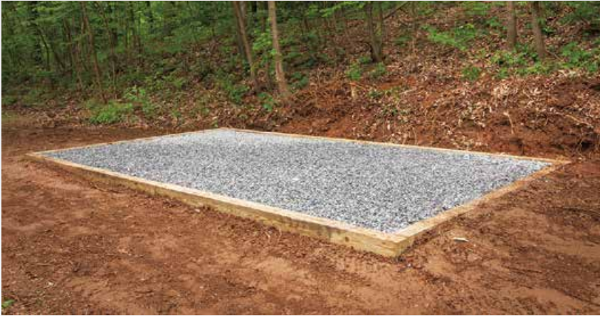
Basic shed pad with pressure-treated wood framing.
